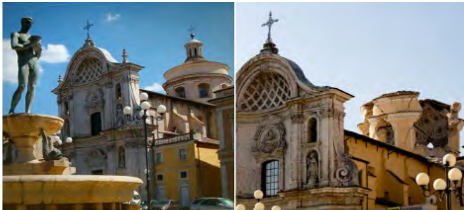
Figure 1.4: Church of Santa Maria del Suffragio, before and after L'Aquila earthquake in 2009, M 5,9 [3].
