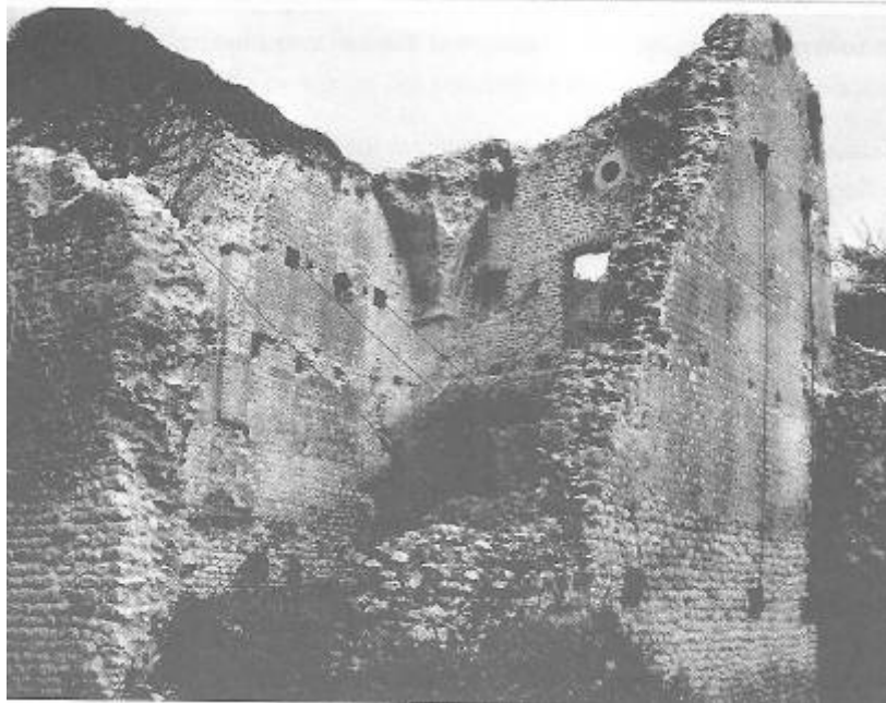
Figure 1.22: Tie-beams for vertical wall in Ninfa – Latina [7].
