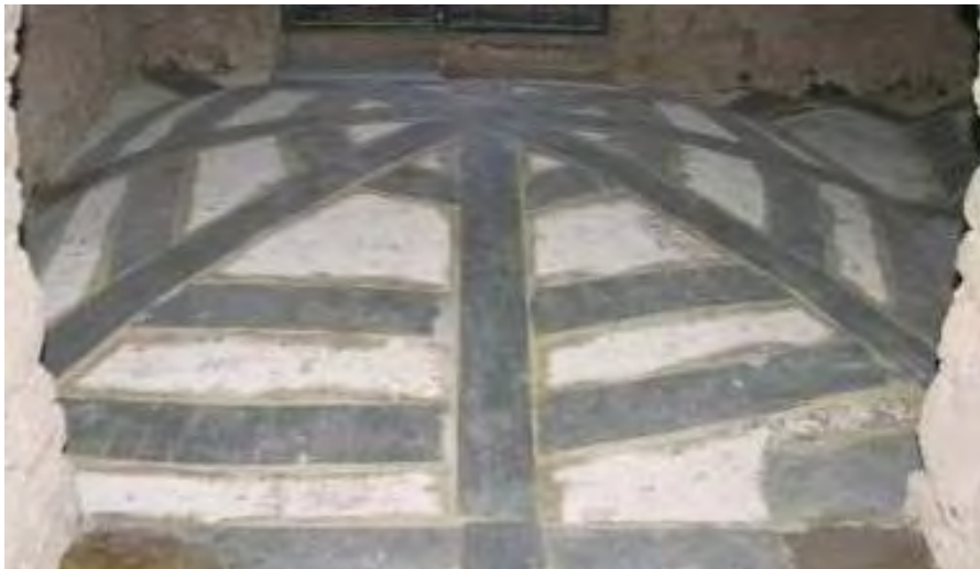
Figure 1.19: Strengthening of a vault with CFRP [3].
